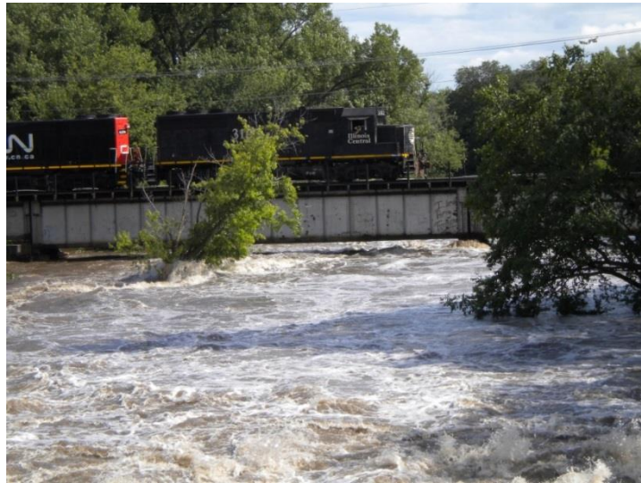
Figure 42. High water levels in the Maquoketa River nearly touching the low-chord of the railroad crossing during the July 2010 flood
